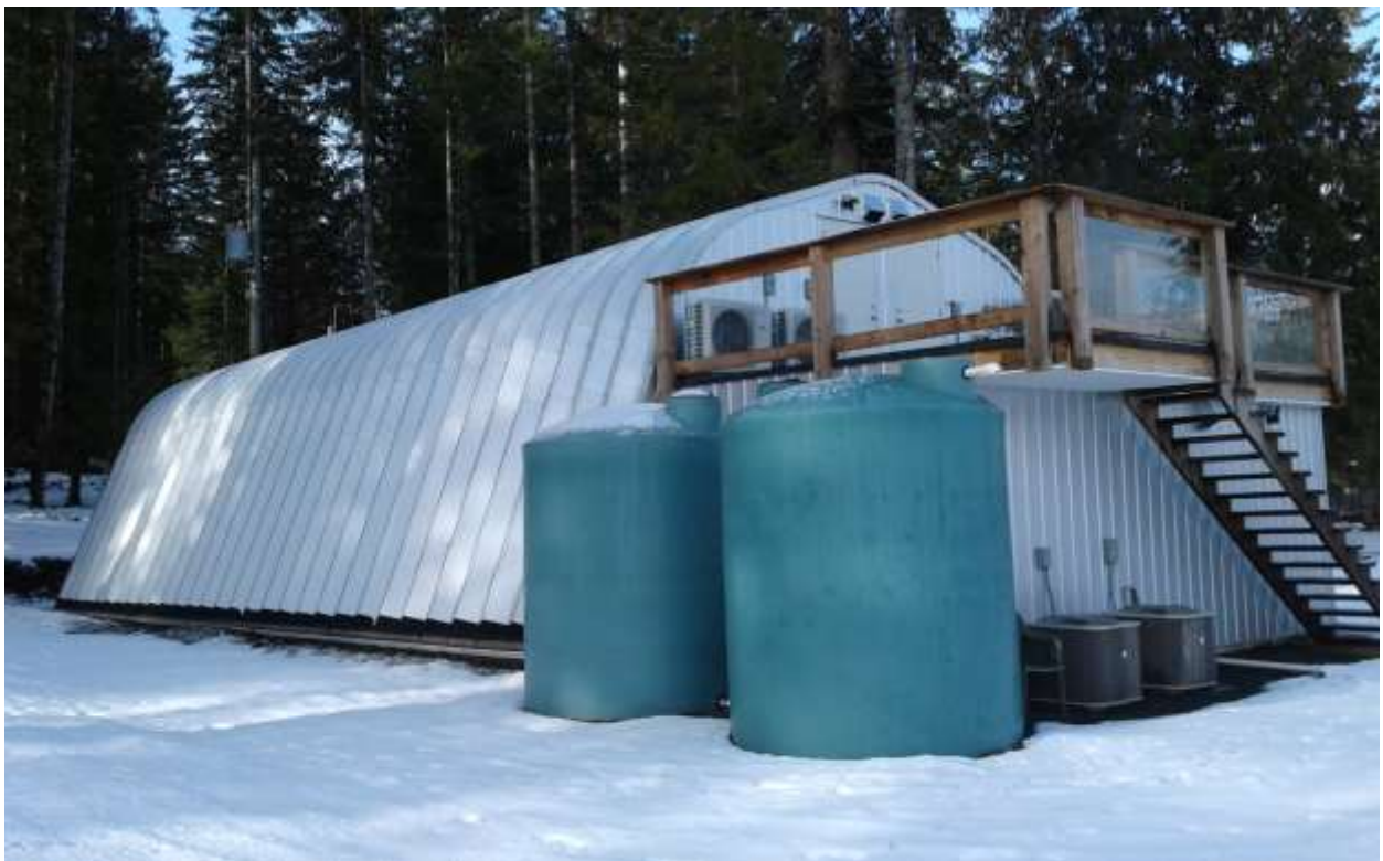
Figure 4: Accessory building, as seen from the rear
